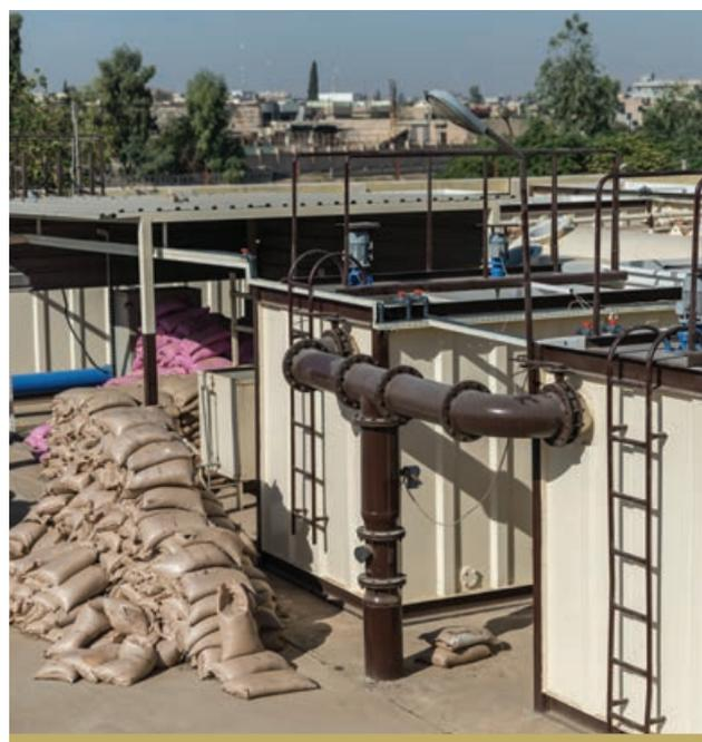
*THE AL SAHIRON WATER TREATMENT PLANT IN EAST MOSUL. FFS WORK IN 2017 TO REHABILITATE THE PLANT, INCLUDING INSTALLING 2 NEW SUBMERSIBLE PUMPS, SEVERAL SUNSHADES AND GENERAL REPAIR WORK, PROGRESSED WELL AND WAS CLOSE TO COMPLETION BY THE END OF THE YEAR. THE AL SAHIRON PLANT, TOGETHER WITH THE AL ZUHOR AND AL SAHIRON PLANTS WILL PROVIDE CLEAN WATER TO 424,800 PEOPLE. ©UNDP IRAQ/CLAIRE THOMAS*
